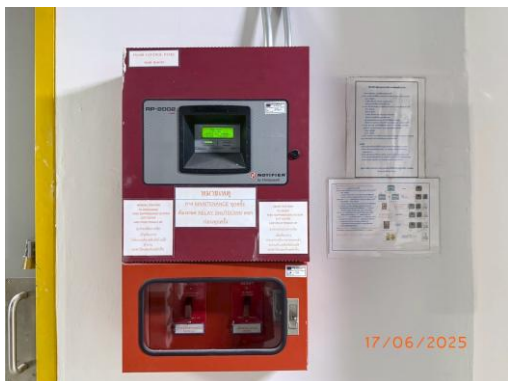
Fire Alarm Control Panel
